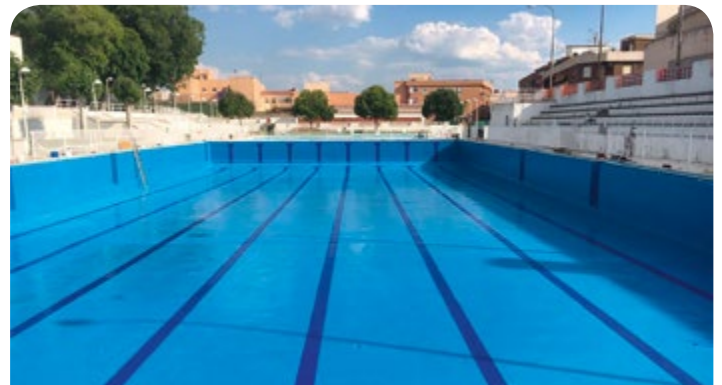
SWIMMING POOLS AND CHEMICAL STORAGE BUNDS
